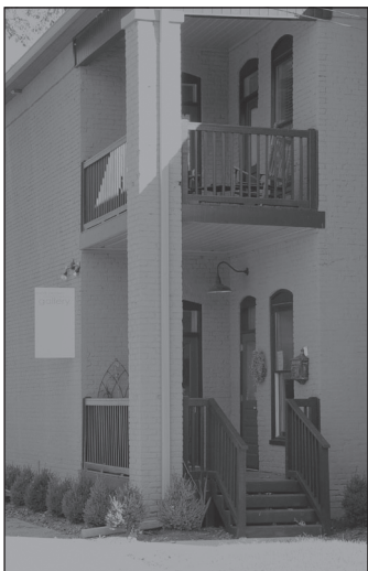
Artist Mark Palmer turned an old, dilapidated building (above) into an attractive gallery (below) when he relocated to Paducah from Washington, D.C.
