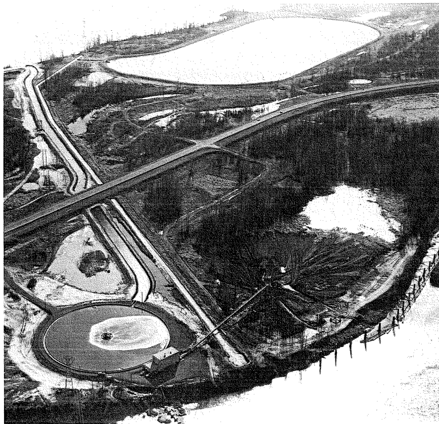
A forest-products mill in Washington has spent close to $20 million on installations such as this to improve water quality control.
