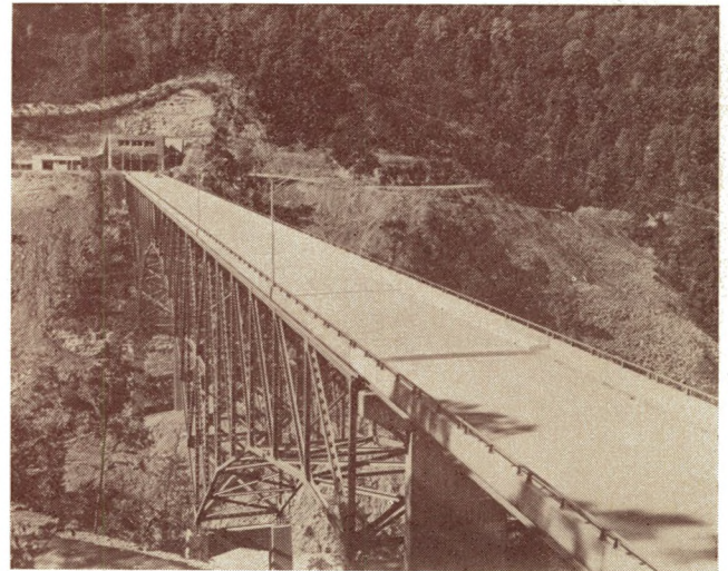
West Virginia Turnpike Commission--The Bender Bridge, highest bridge east of the Mississippi River, is named in honor of Congressional Medal of Honor winner Sergeant Stanley Bender. The entrance to the Memorial Tunnel is shown in the background.
