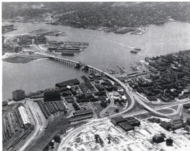
Elizabeth River Tunnel Commission—Elizabeth River Bridge, Norfolk, with tunnel entrance in left background.
