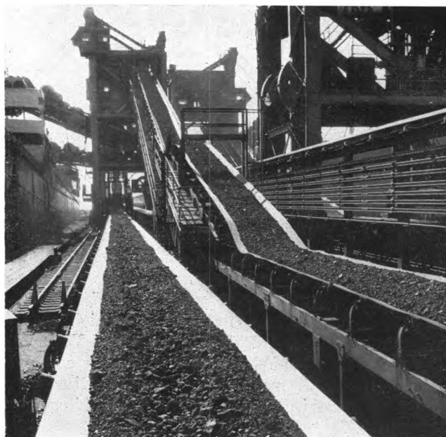
—Through the courtesy of the League of Virginia Counties A close-up of the multiple conveyor system on the C. & O. pier 14 at Newport News.
