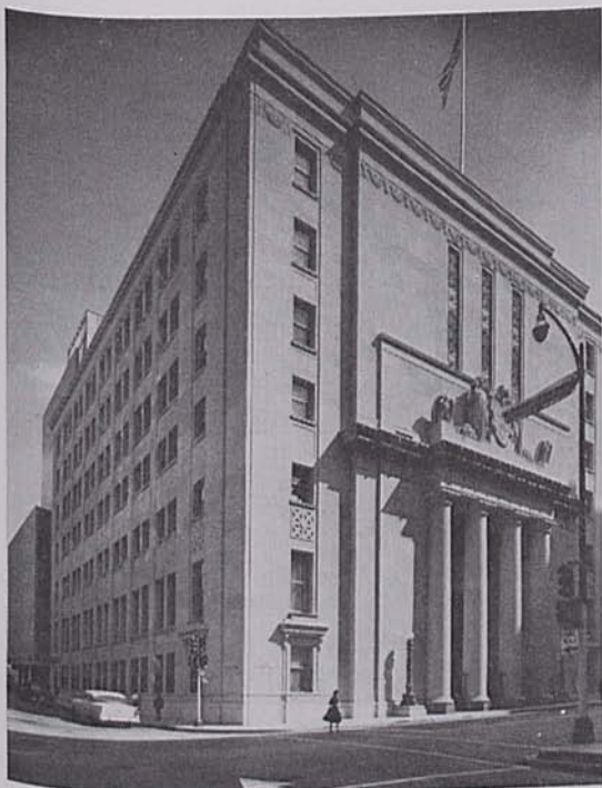
Head Office Building of the Bank. View shows front of old building, after remodeling, and new addition at rear. Enlargement and remodeling completed in fall of 1960.
