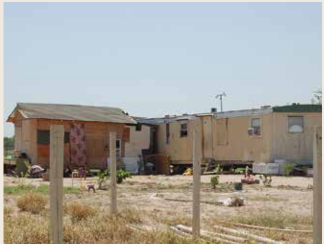
These are “hybrid” colonia homes—an RV or mobile home with a wooden or cinder block structure attached. Photo credit: Federal Reserve Bank of Dallas
