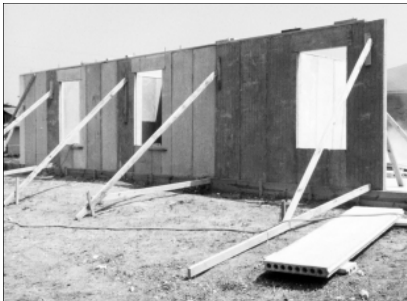
Fibrecrete panels replace more costly, traditional wood frames.
