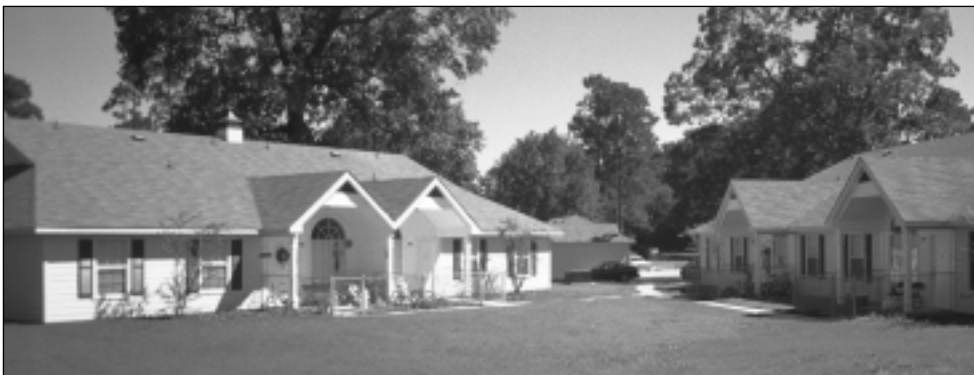
Using tax credits, developers can provide affordable rental housing like these attractive homes in Dayton Park, Dayton, Texas.
