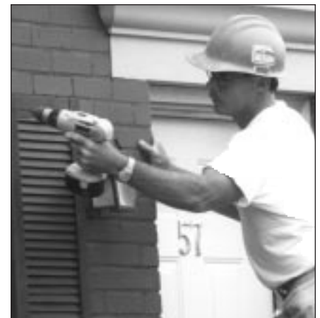
Adding the finishing touches....
