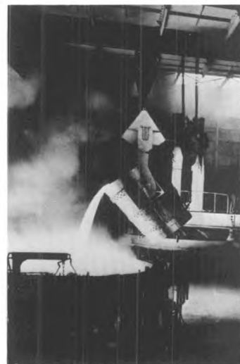
An electric steelmaking furnace receives a charge of molten iron from blast furnaces.
