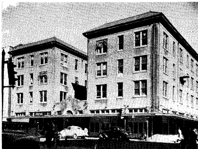
The Meaher office building located at the corner of St. Michael and St. Joseph Streets, in Mobile, Alabama, is the first major nonresidential structure to be leased by the Government for conversion into housing facilities. Remodeling will require only minor structural alterations to yield 200 dormitory units for use in one of the country's most critical housing situations.
