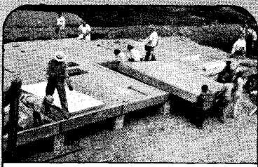
1:15 p. m. . . . With three workmen at either end of a floor section, it is easily lifted.
