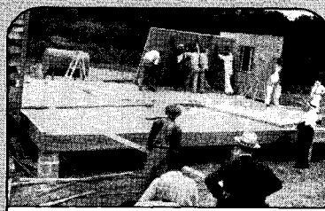
1:25 p. m. . . . Wall sections are put in place as soon as the flooring is fastened down.
