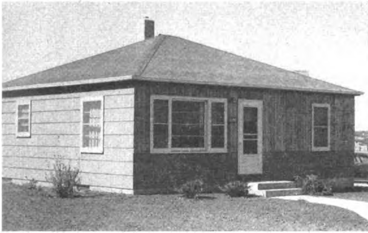
One of the 4 basic house designs used in Bel Aire Addition.
