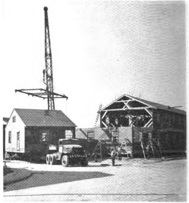
The third step is to load the section on a special trailer and haul it to the site
