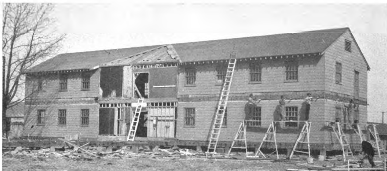
The first step in converting a barracks building into a house is to cut off the second floor
