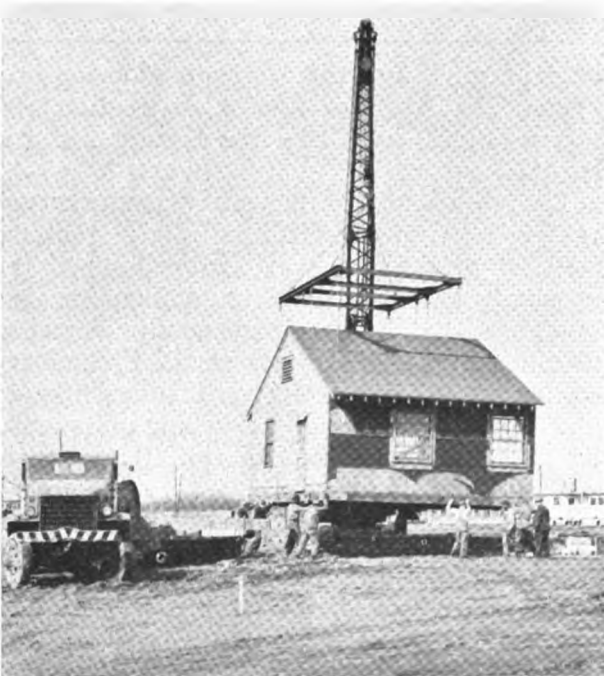
The fourth step is to take the section off the trailer and put it on its foundation
