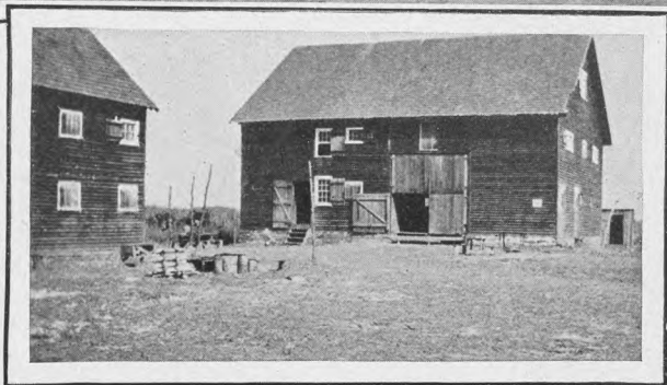
HOUSES FOR WORKERS ON LARGE TRUCK FARM, SOUTHERN NEW JERSEY SHANTY HOUSING 47 PERSONS, SOUTHERN NEW JERSEY
