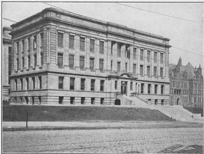
CHILDREN'S BUILDING (JUVENILE COURT AND DETENTION HOME), ST. LOUIS, MO.
