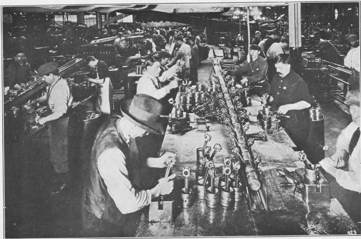
PLATE XIX.—PISTON AND CONNECTING-ROD ASSEMBLY. BENCH WORK.
