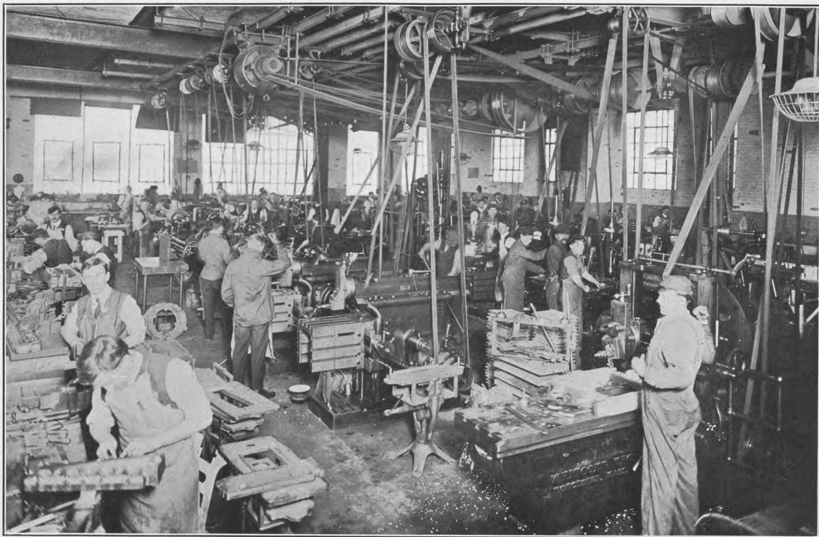
PLATE VII.—MACHINE SHOP. PLANER IN FOREGROUND AT RIGHT, SHAPERS NEXT; BENCH WORK AT LEFT.
