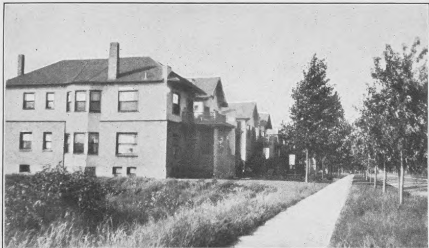
PLATE III.—EXCEPTIONALLY GOOD COMPANY HOUSES IN AMBRIDGE.
