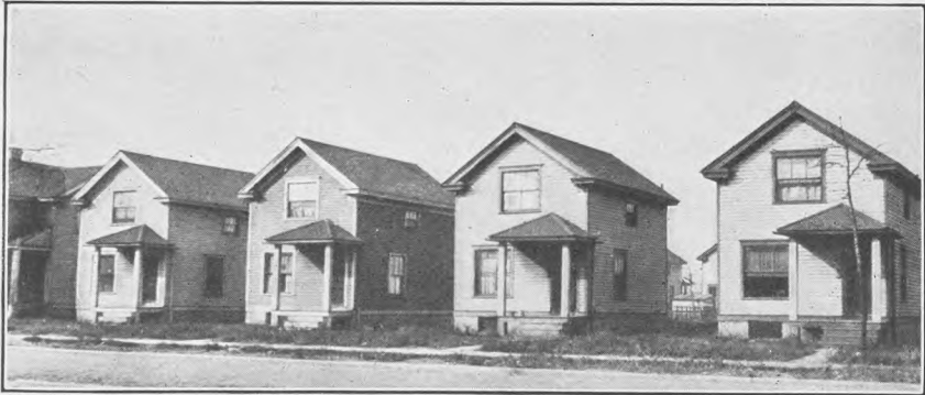
PLATE II.—COMPANY HOUSES OF THE OLDER TYPE.
