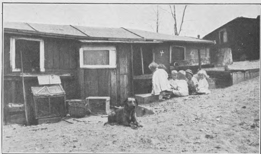
PLATE X.—A SHACK OF MAKESHIFT CONSTRUCTION.
