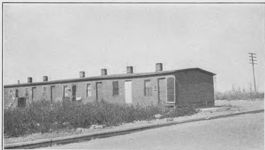
PLATE VI.—A ONE-STORY FRAME SHACK.
