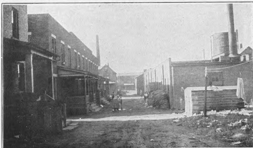
PLATE X.—PUMP AND GARBAGE VAULT.
