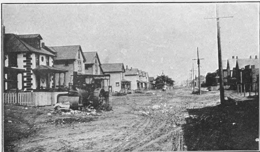
PLATE VI.—UNPAVED STREET ALWAYS WET.
