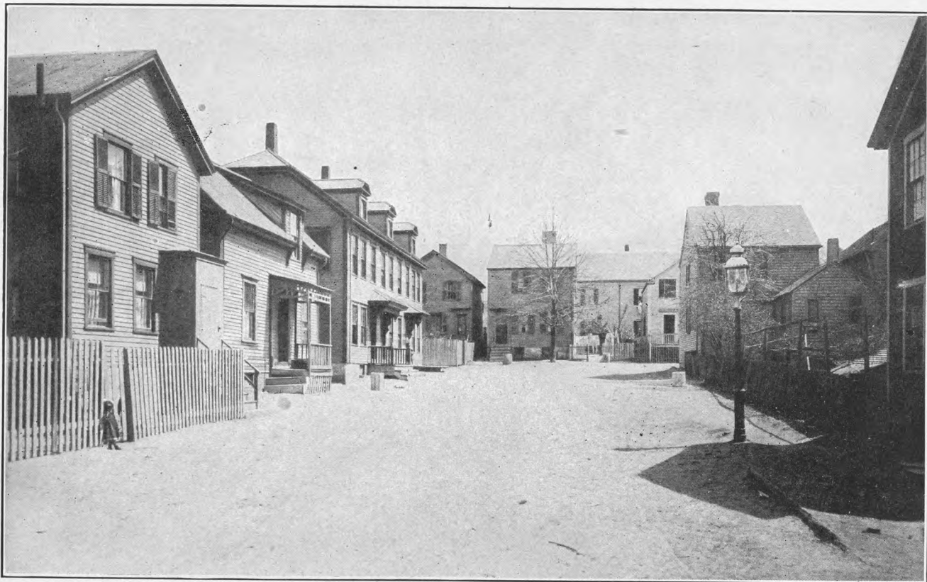
PLATE IX.—VIEW IN THE CENTER OF THE NATIVE BLACK SECTION; HERE THERE IS NO PAVING, AND PRIVIES ARE FOUND IN THE YARDS.
