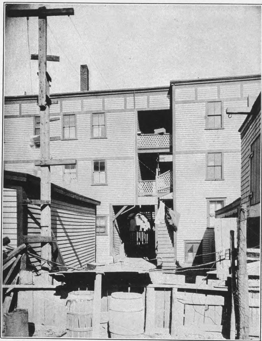
PLATE XIII.—ANOTHER WAY OF COMPLYING WITH THE FIRE REGULATIONS— TWO TENEMENTS USING A SINGLE BACK EXIT.
