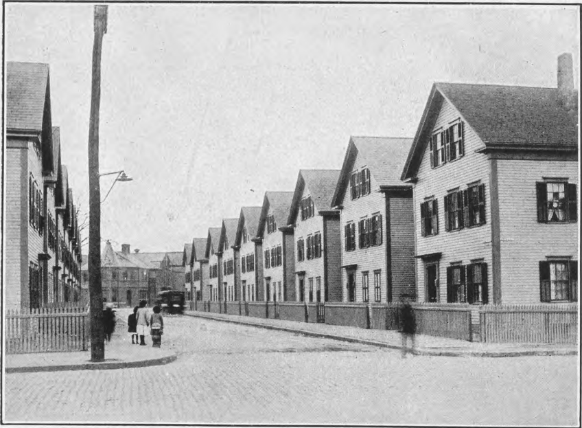
PLATE III.—PART OF A GROUP OF 27 MILL HOUSES—TOILET ADJOINING THE KITCHEN IN EACH APARTMENT.
