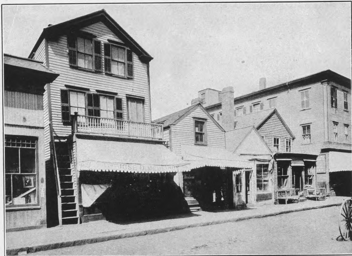
PLATE XII.—METHOD OF MEETING THE FIRE REGULATIONS WHICH REQUIRE TWO EXITS—ALMOST PERPENDICULAR STAIRS ON THE FRONT OF THE HOUSE.
