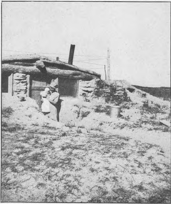
THE FATHER OF THIS BABY HAS TAKEN THE PRECAUTION OF FENCING THE ROOF OF THE DUGOUT AGAINST CATTLE.
