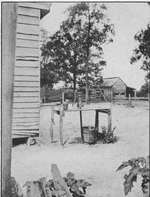
PLATE XII.—DRILLED WELL CONVENIENTLY NEAR THE HOUSE.
