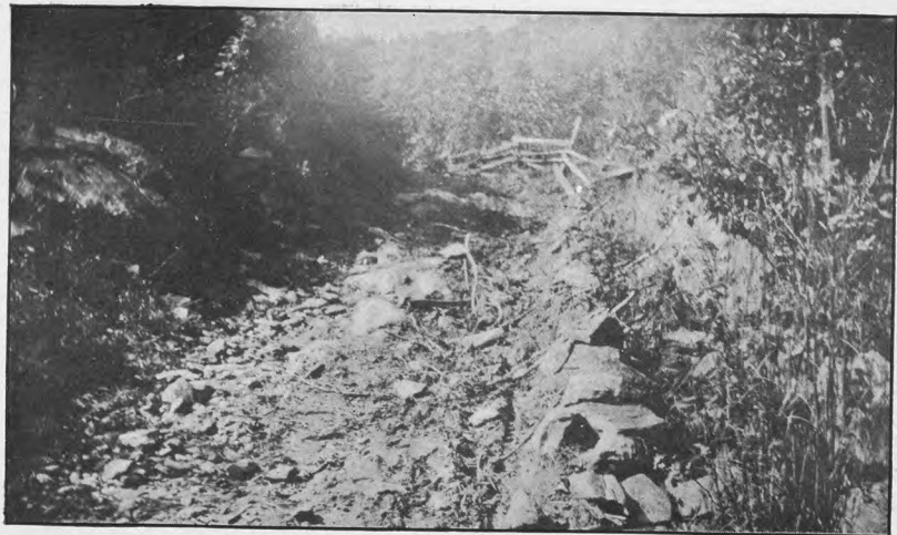
PLATE XXI.—BAD ROADS—AN OBSTACLE TO PROGRESS.
