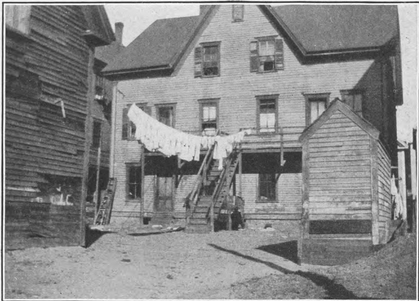
PLATE V.—FOUR-FAMILY HOUSE, CONTAINING FOUR DARK BEDROOMS. TOILETS IN YARD.
