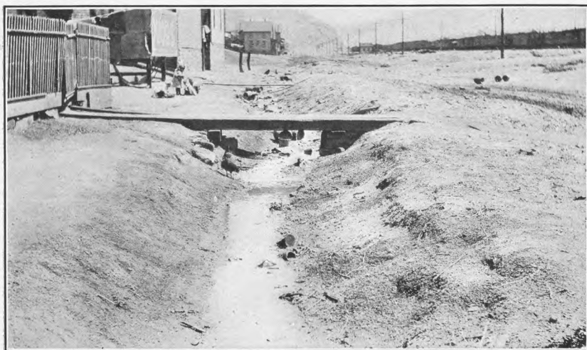
VIEW OF AN OPEN DITCH ON PLUM STREET, WHICH RECEIVES HOUSE DRAINAGE OF ALL KINDS.
