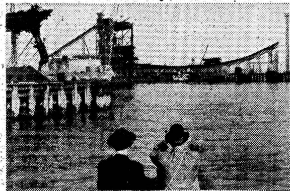
At Newport News, Va., C&O's Atlantic port, Mr. Price inspects the new coal export pier, just completed. Almost half of overseas export coal is handled here. He also saw the new $8 million pier designed to unload 60 tons of import ore per minute.
