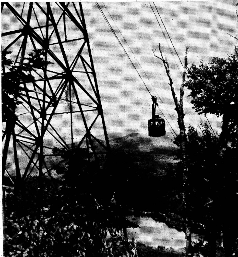
You'll Float Through The Air—For A Mile. This is a cable tramway for tourists that goes up Cannon Mountain at Franconia Notch in New Hampshire. The heavy wire ropes are well over a mile long, 1 1/8 inch in diameter and they weigh 28 tons apiece. The cable was made and installed by American Steel & Wire Division of United States Steel.
