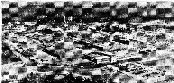
Chemstrand Corporation's multi-million dollar nylon fibre manufacturing plant near Pensacola, Florida, is one of the many industries newly located along the L&N.
