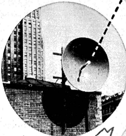
4. A similar antenna receives the picture at the LaSalle Street Union Station and feeds it to another monitor there.
