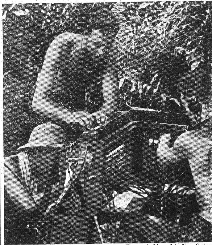
U. S. Army Signal Corps installing switchboard in New Guinea
