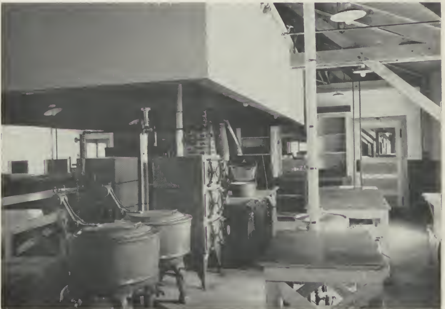
FIGURE 147: Ready to begin service this modern, well-equipped kitchen is attached to the hospital unit at Heart Mountain Relocation Center.
