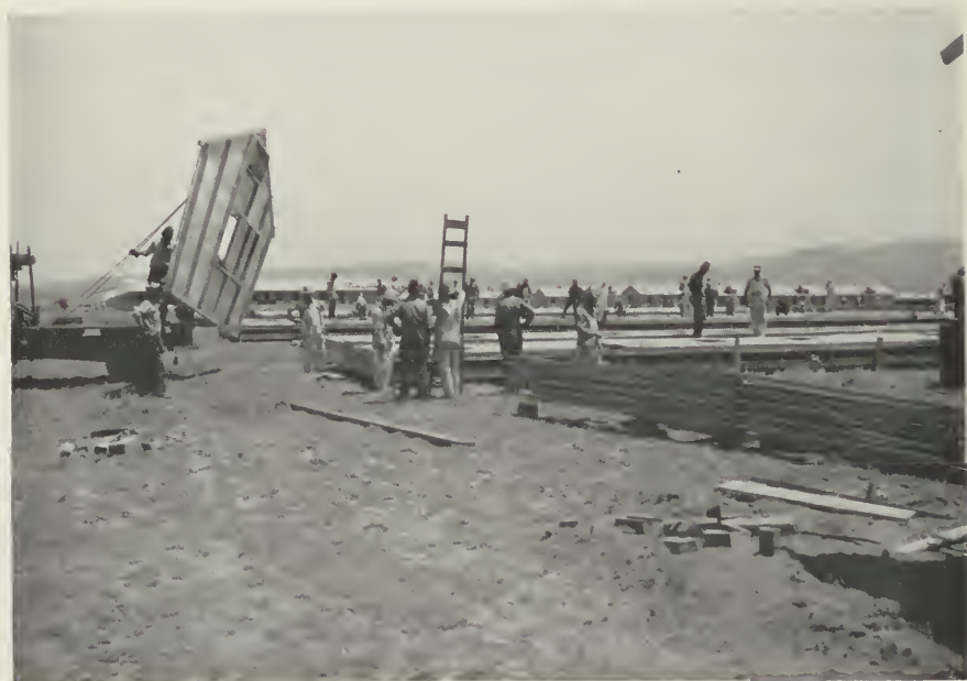
FIGURE 143: Buildings were put together in sections in a central construction area and these sections hauled by truck to the building site.
