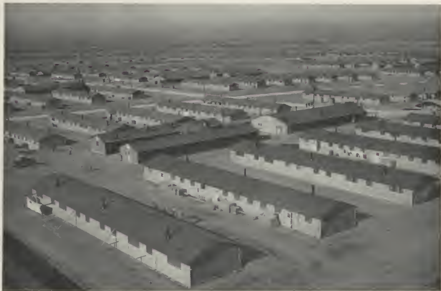
FIGURE 145: Panorama of Granada Relocation Center, Amache, Colorado, showing in the foreground a typical barracks unit consisting of 12 six-room apartment barracks buildings, a recreation hall, laundry and bathhouse, and the mess hall, constructed by Army Engineers. The Center is made up of 30 such blocks, complemented by hospital buildings, administrative office buildings, living quarters, general warehouse structures and Military Police quarters.
