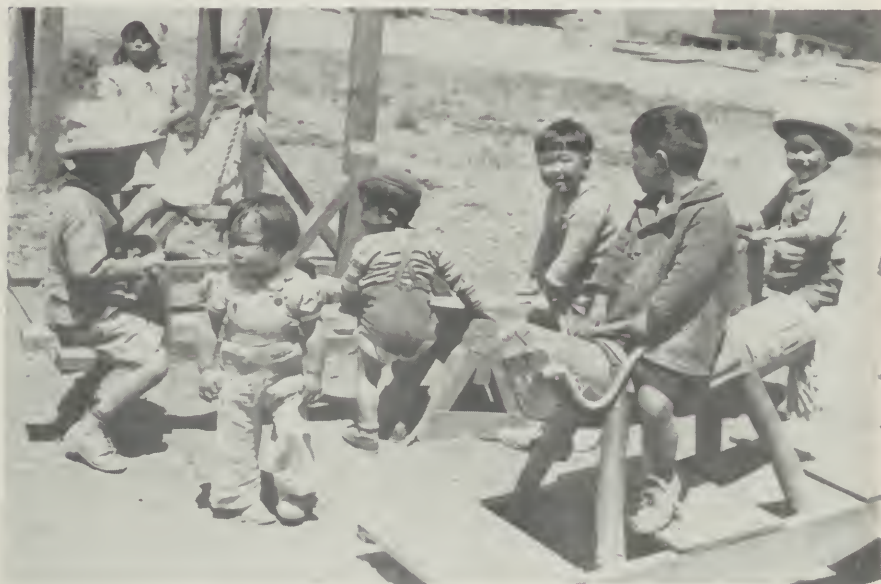
FIGURE 73: A play scene at Tanforan (California) Assembly Center, with home-made rocking horses, teeter-totters, and swings. Playfields with rustic equipment made of scrap material and other installations stimulated recreational and outdoor play activities which many young evacuees had never before enjoyed.
