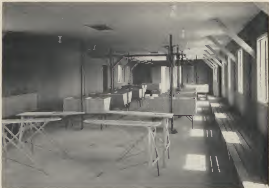
FIGURE 148: Airy and spotless is this section of a Relocation Center laundry with modern plumbing and tanks, ironing boards and side-wall bench for bundles.
