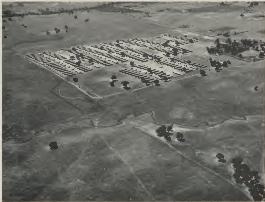
FIGURE 16-i—SACRAMENTO ASSEMBLY CENTER
