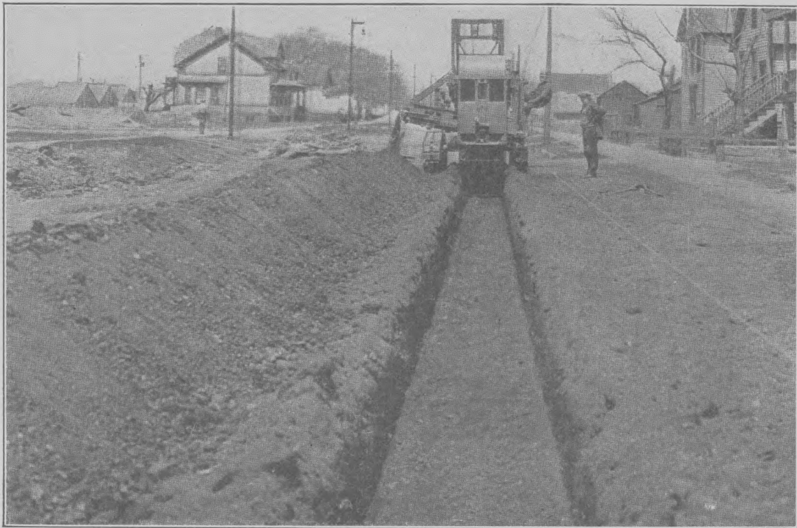
FIGURE 2.—CURB AND GUTTER DITCHER. ON JOB SHOWN, MACHINE REPLACED GANG OF 50 MEN
