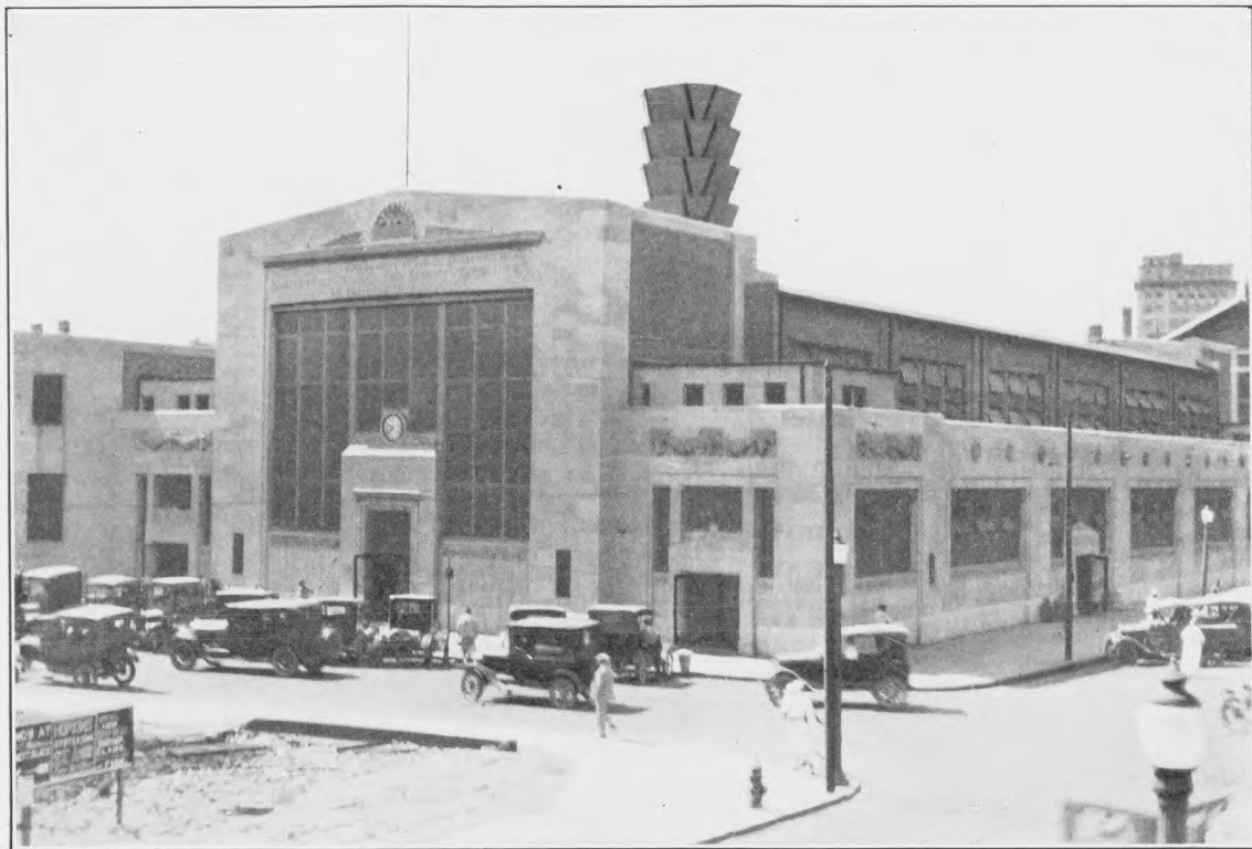
EXTERIOR OF MUNICIPAL MARKET BUILDING, NORFOLK, VA.
