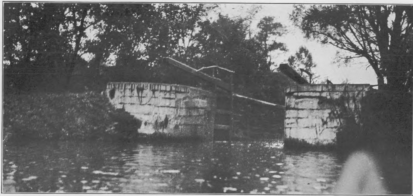
FIG. 1.—LOCK WITH SWINGING GATES.
