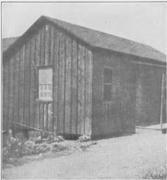
FIG. 4.—An old-style board and batten 3-room miner's cottage still in use in an isolated mining town of Pennsylvania.
