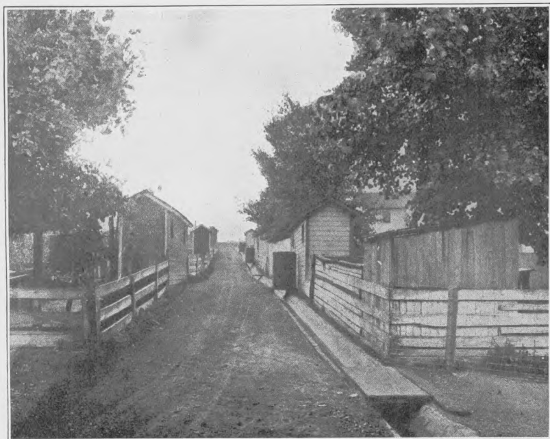
FIG. 5.—Improved alley in coal and coke town in western Pennsylvania. Note drainage gutter with garbage receptacles over it.
