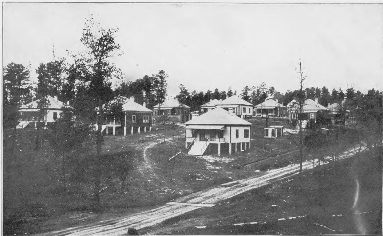
FIG. 6.—New coal mining camp, Birmingham (Ala.) district, constructed in 1916. Houses built before grading and laying of streets. All cottages of similar plan and adapted for conversion into double houses. Used as 1-family 4-room houses. Running water in kitchen; electric light. Ceiled inside; composition roof.
