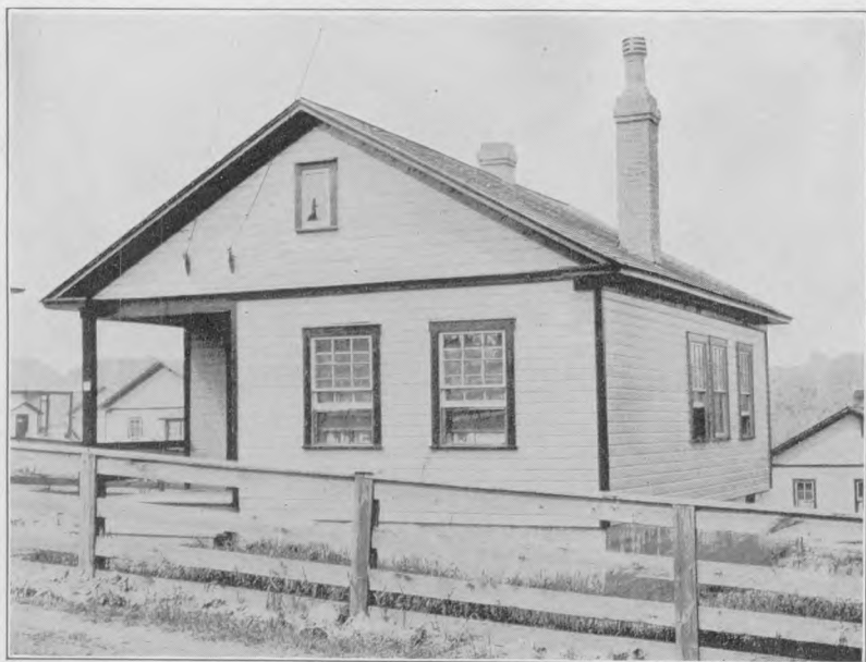
FIG. 7.—Miner's cottage in an Ohio town. Four rooms; rent $10 per month. Cost in 1912, $675. Electric lights, but no modern sanitary improvements. Better than the average.
