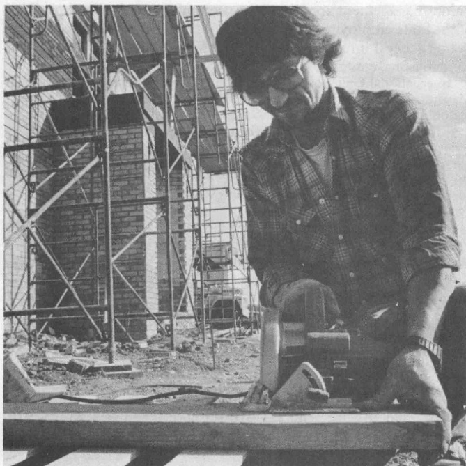
Carpenters must be very careful when operating power equipment.
