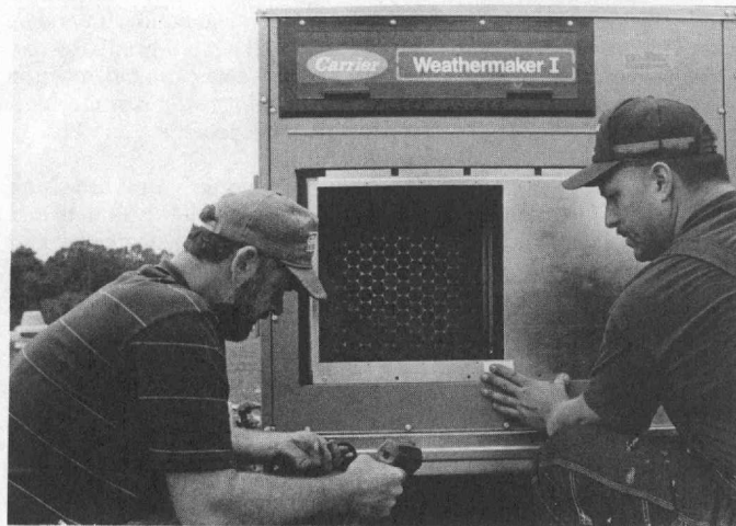
Air-conditioning mechanics diagnose the problem and make repairs.
