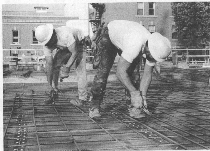
Reinforcing workers work together to tie-wire reinforcing bars.
