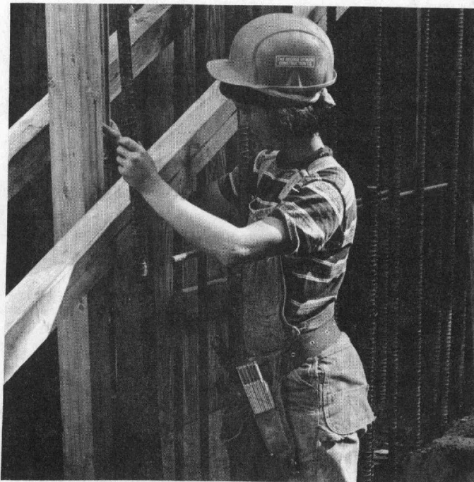
Carpenters use levels to check the accuracy of their work.
