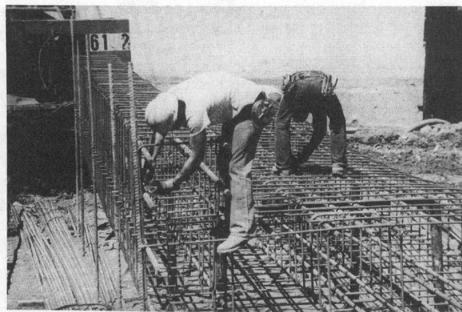
Reinforcing iron workers work together to wire-tie reinforcing bars.
