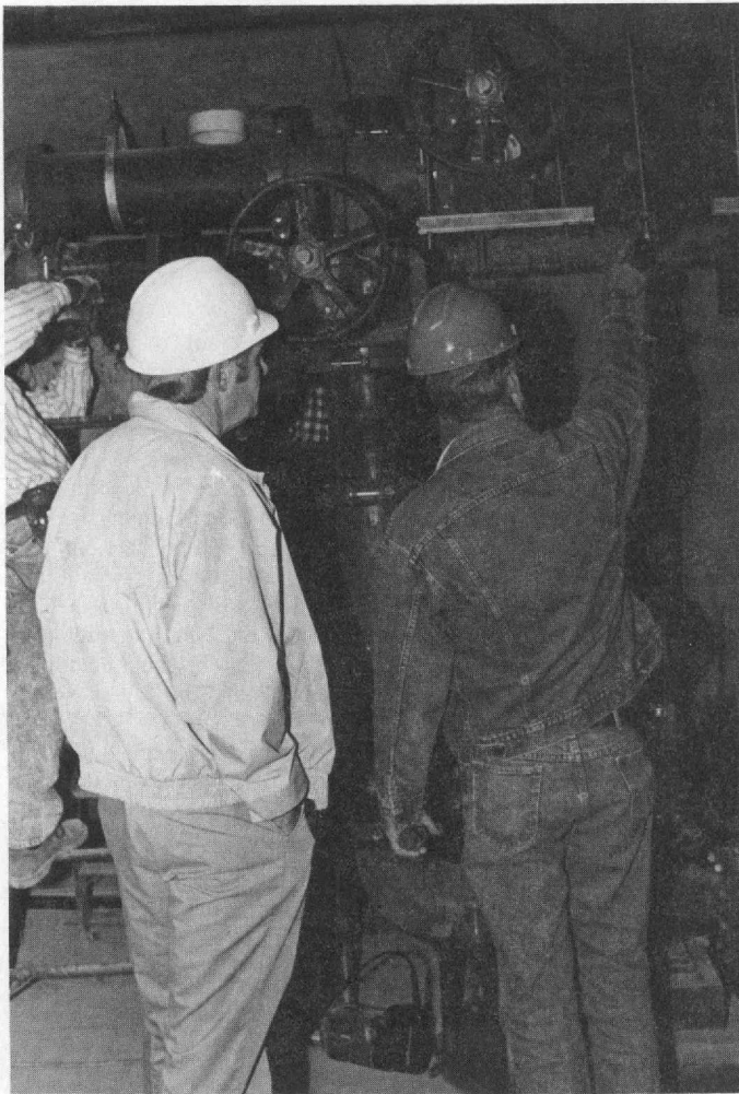
Building inspectors monitor the installation of piping.
