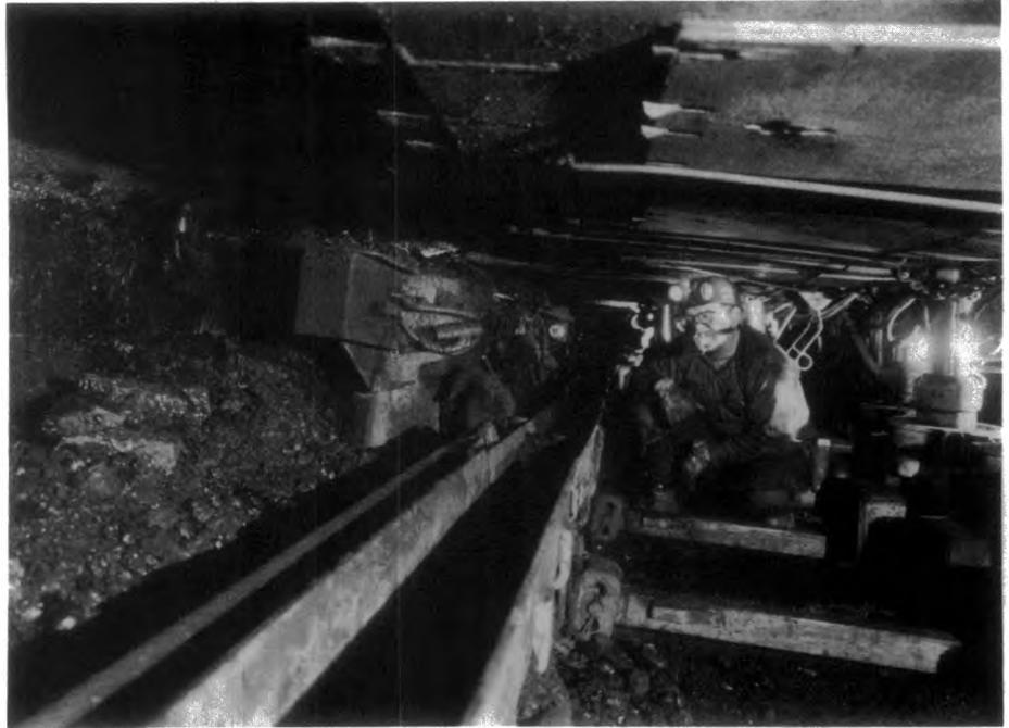
Hydraulic jacks support the roof as the coal is sheared from the face of a seam.
