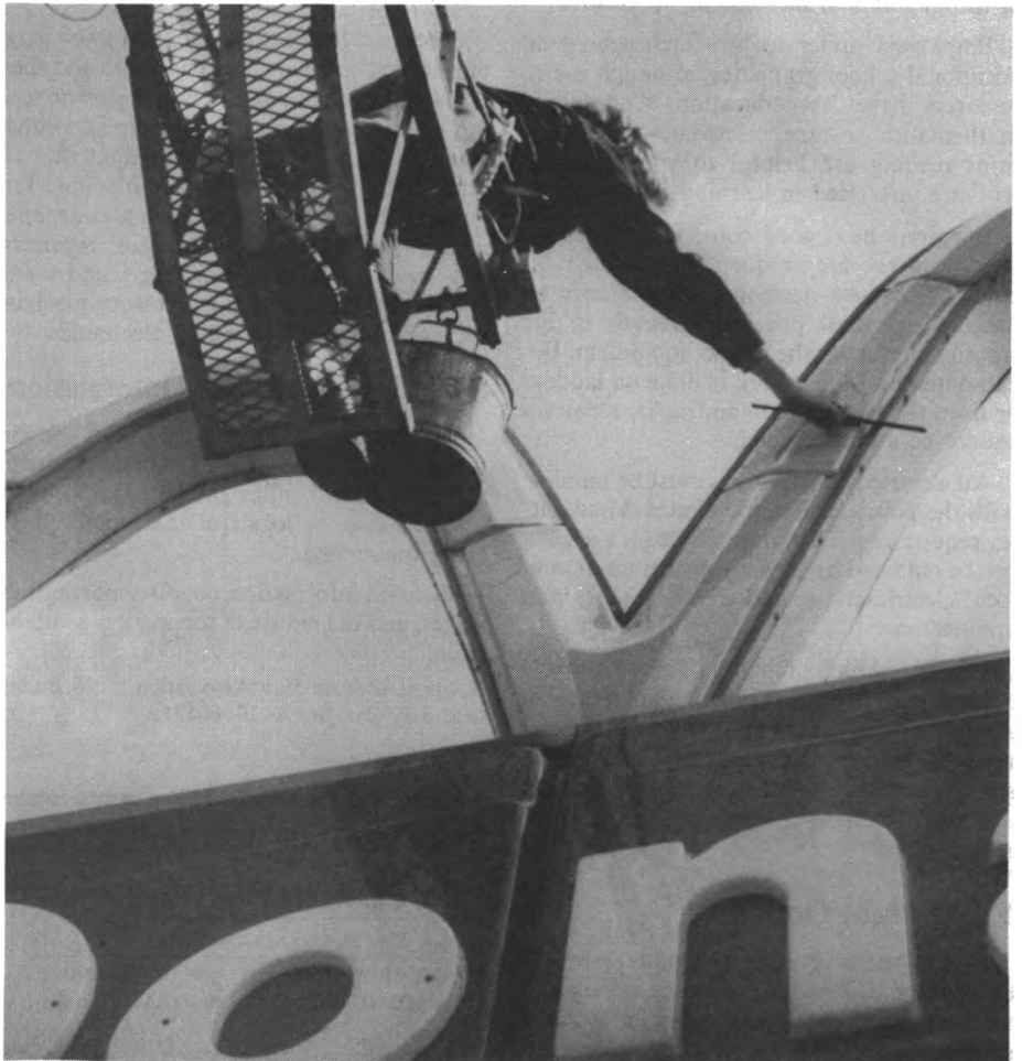
Repairers often work on boom cranes to reach tall signs.
