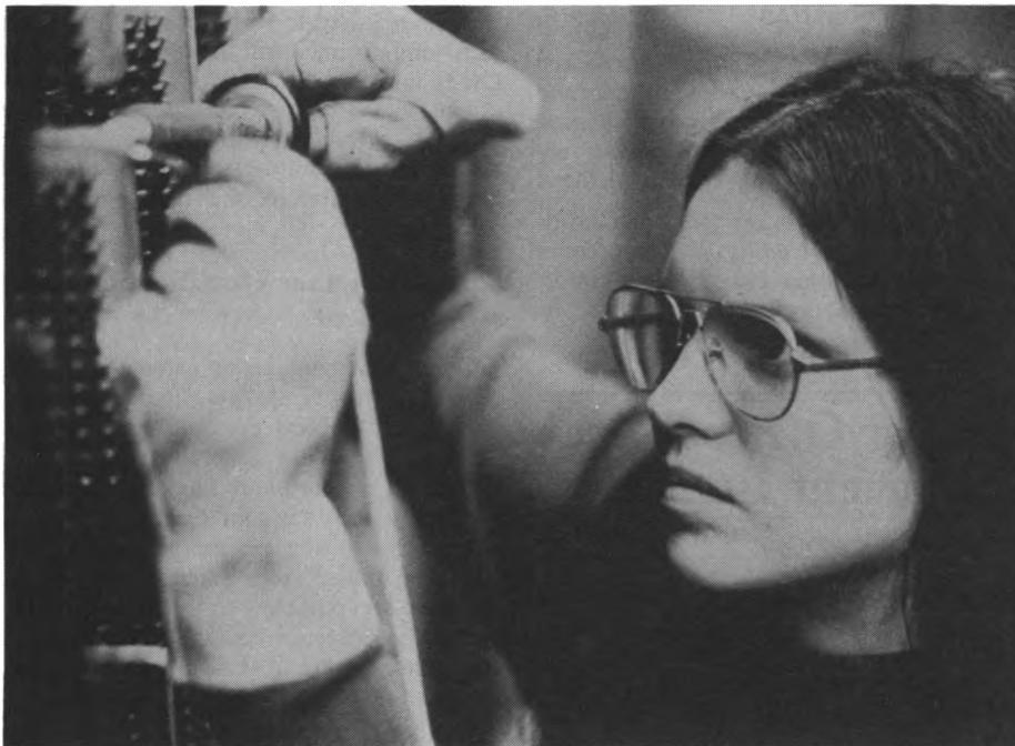
Frame wirer solders a pair of wires to a set of terminal lugs.
