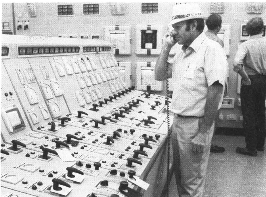
Following orders of load dispatchers, operators regulate the flow of electricity onto various powerlines according to the changing needs of customers.
