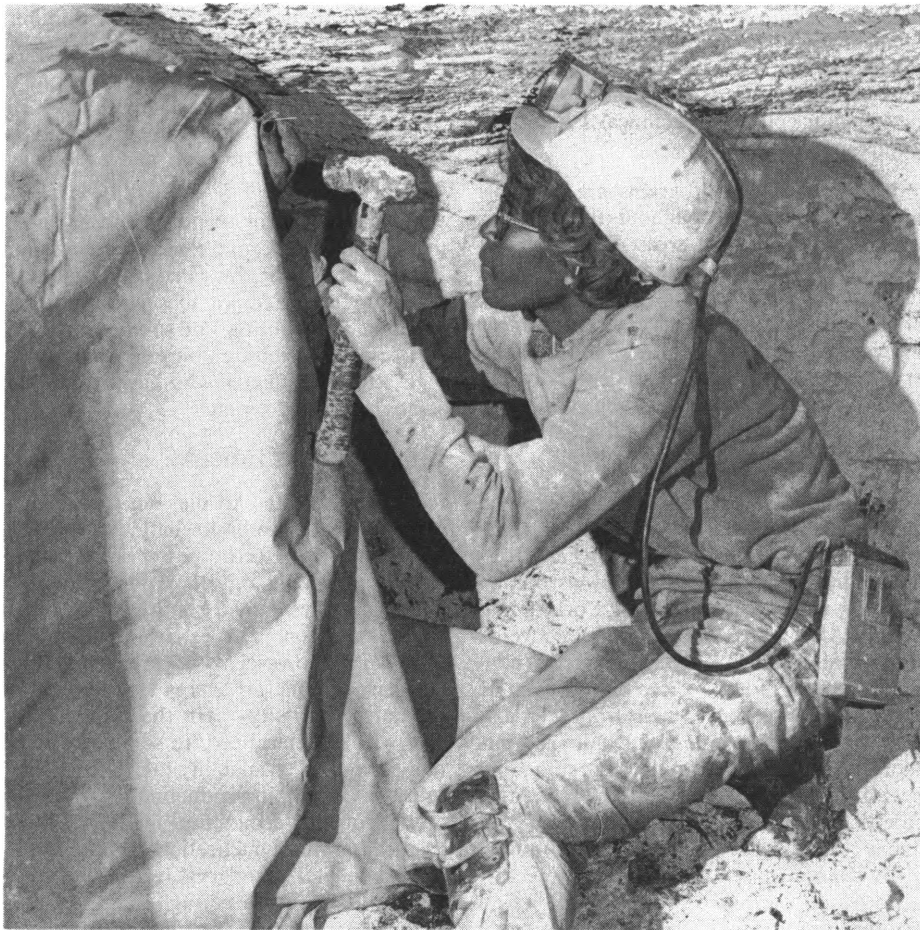
Miner fastens a brattice cloth, which helps control ventilation underground.
