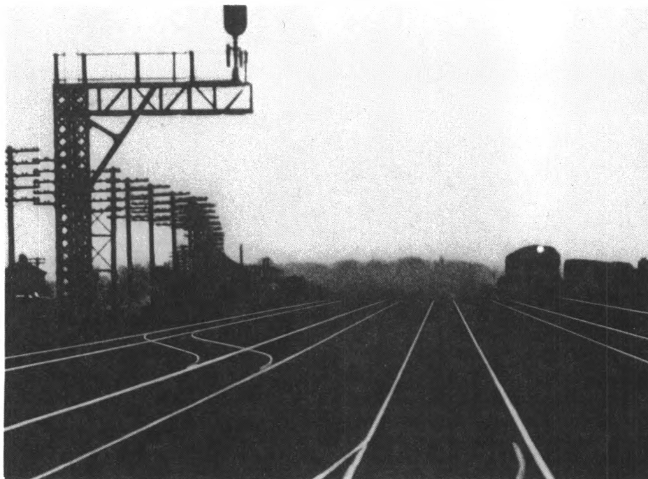
Trains are one of the most efficient methods of transporting large amounts of freight over long distances.
