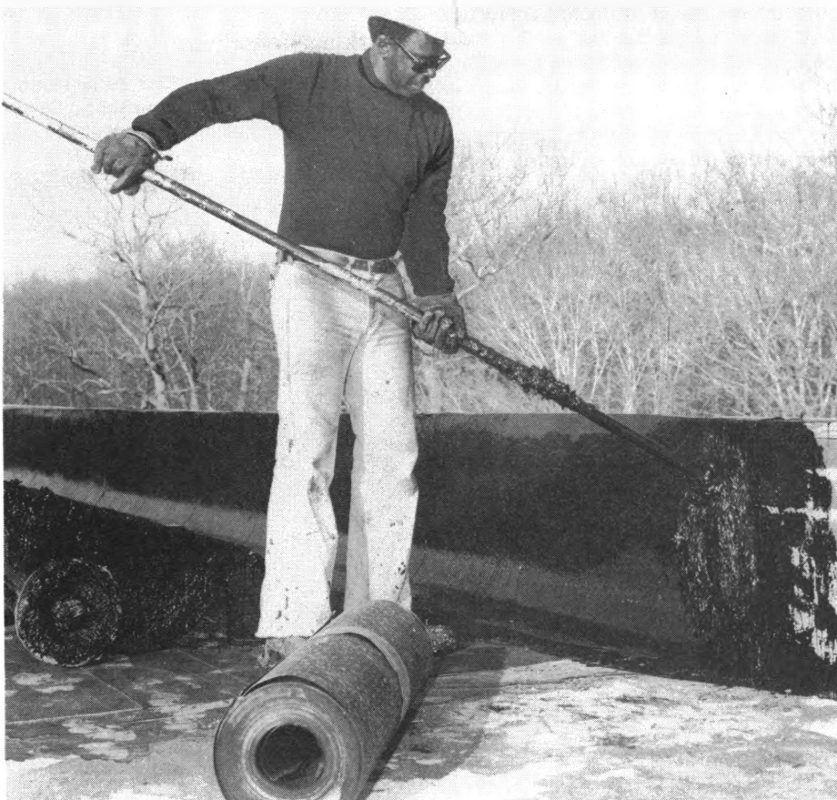
Roofers often work with hot, sticky substances such as tar.
