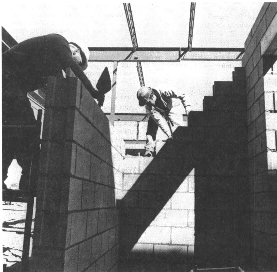
Bricklayers leveling and aligning freshly laid cement block.
