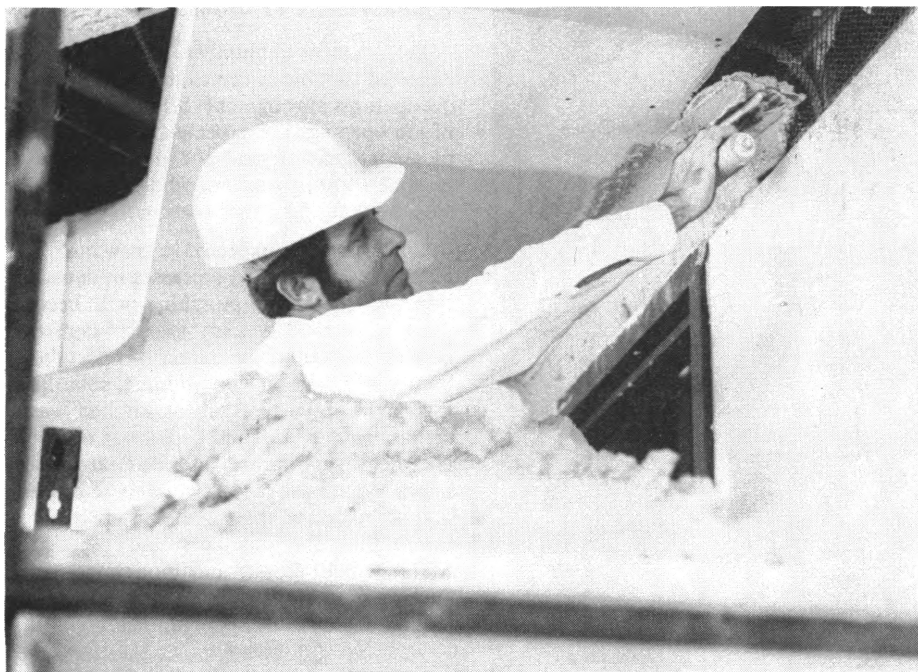
Plasterer applies scratch coat onto base molding.
