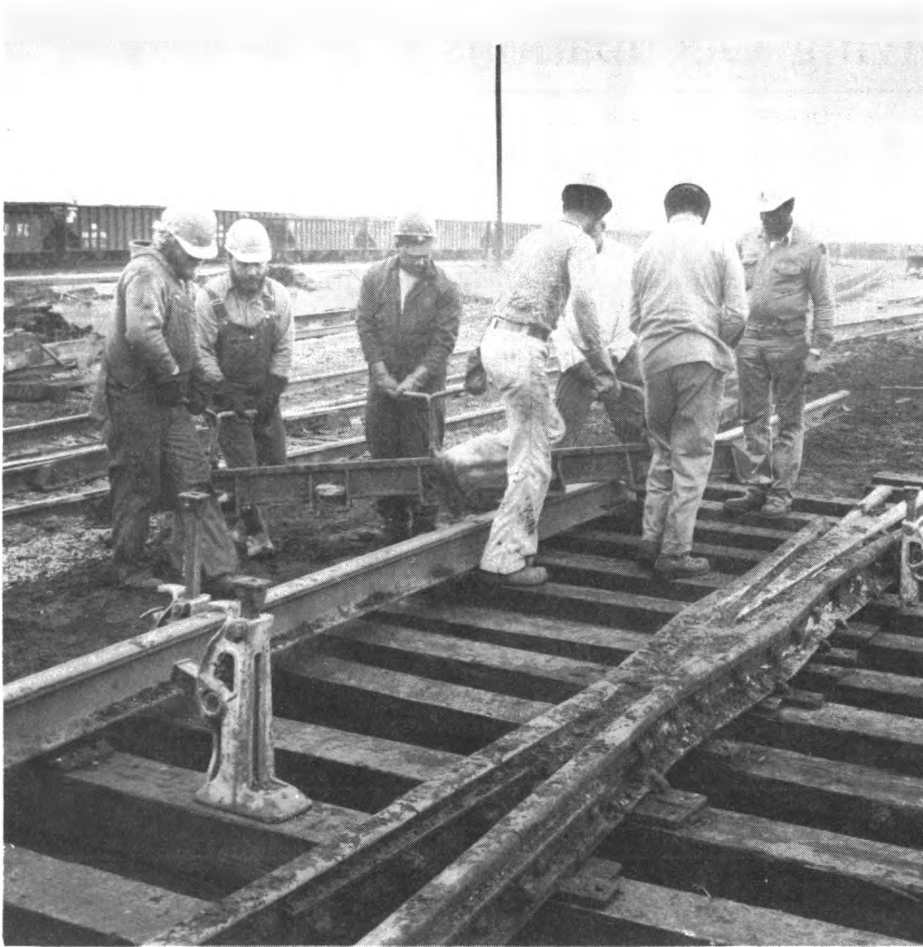
Laying track is a strenuous job.
