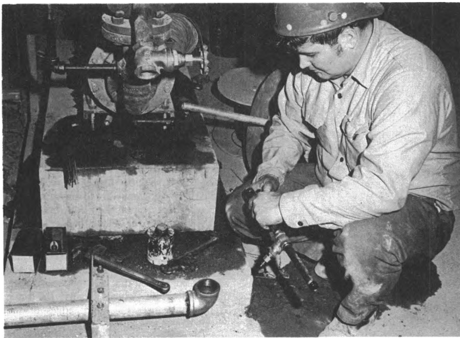
Plumbers repair as well as install pipe systems.
