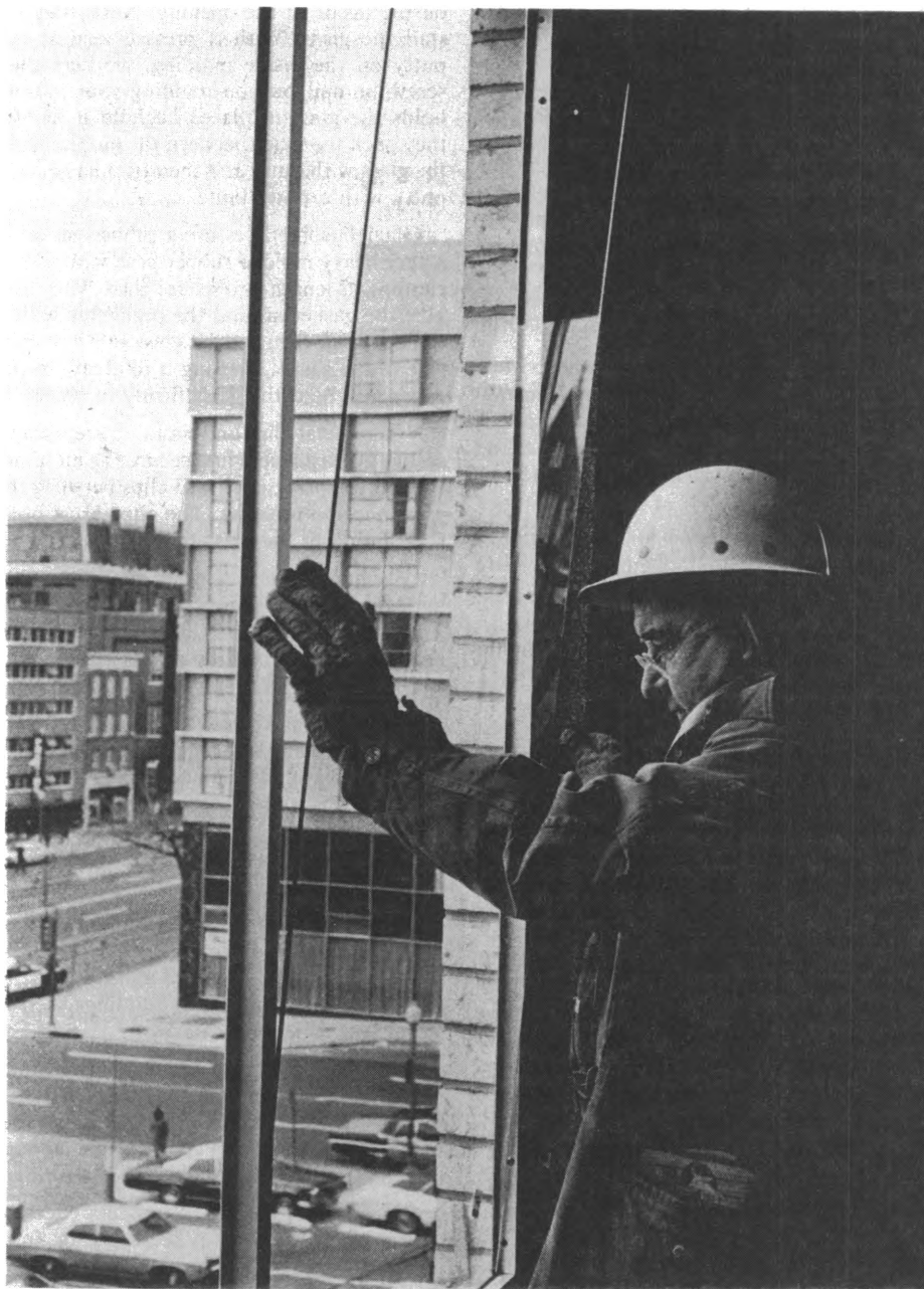
Glaziers often set glass in place by hand.
