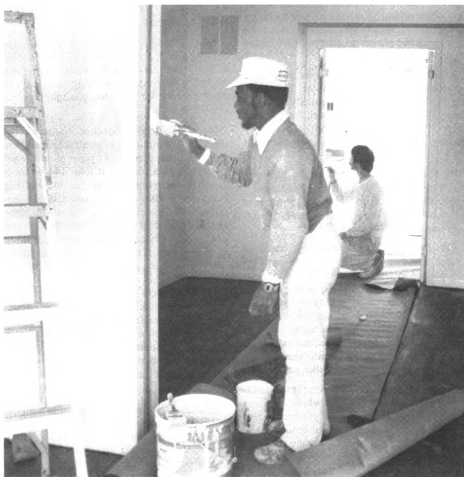
Painters must work quickly and neatly.
