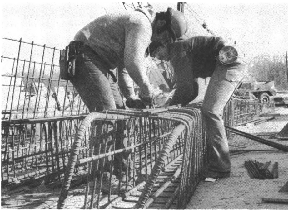
Ironworkers assemble rods that will be used in making concrete pillars.
