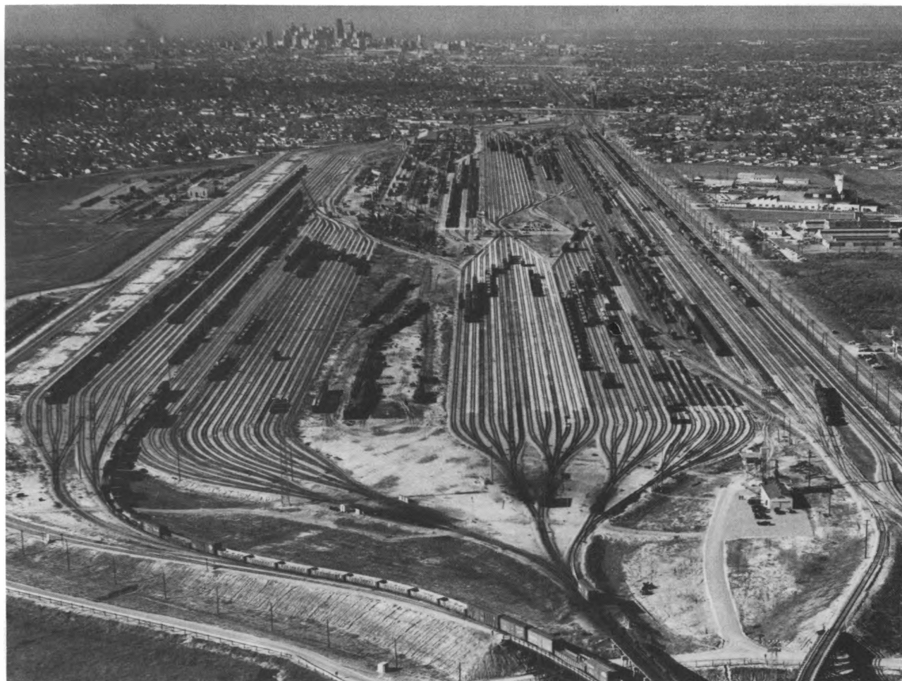
The Nation's 200,000 miles of railroad track are an important means of moving people, food and industrial goods.
