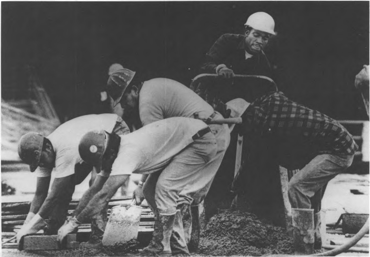
Laying concrete is a team effort.
