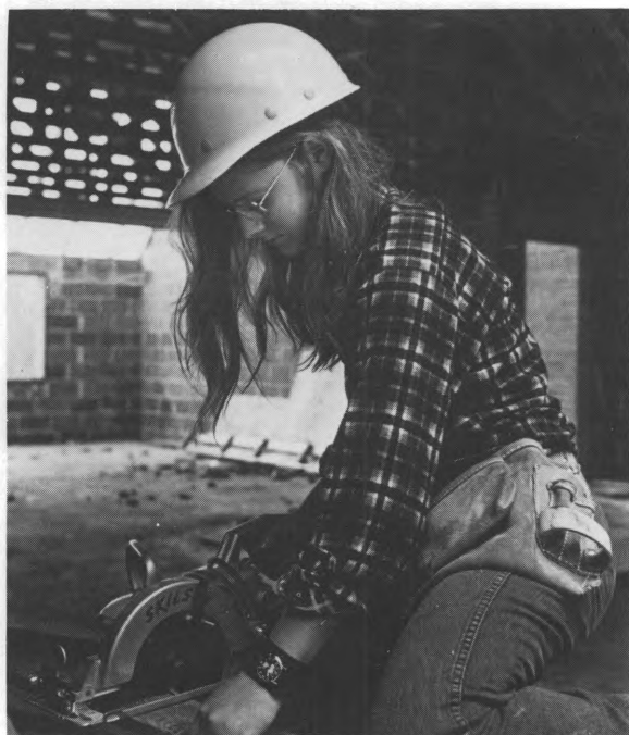
Carpenters work quickly and accurately with hand tools or power tools.
