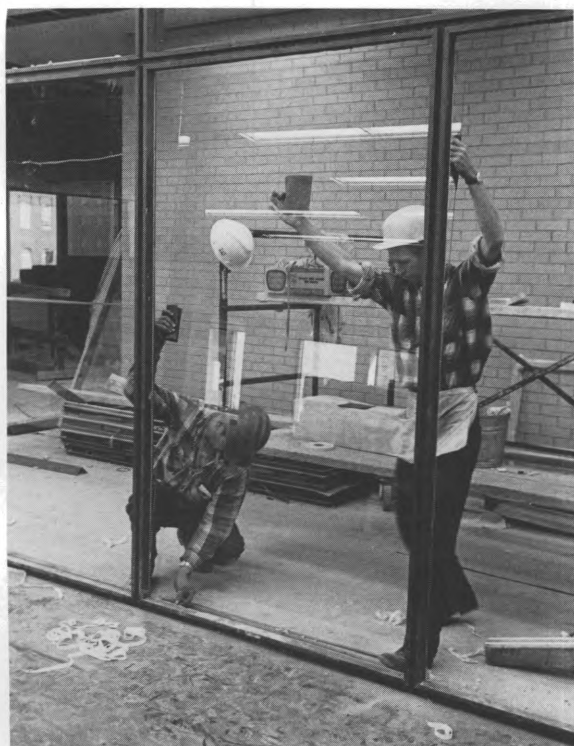
Glaziers install all types of building glass.
