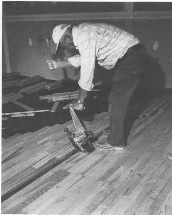
Years of experience enable this floor installer to work quickly.
