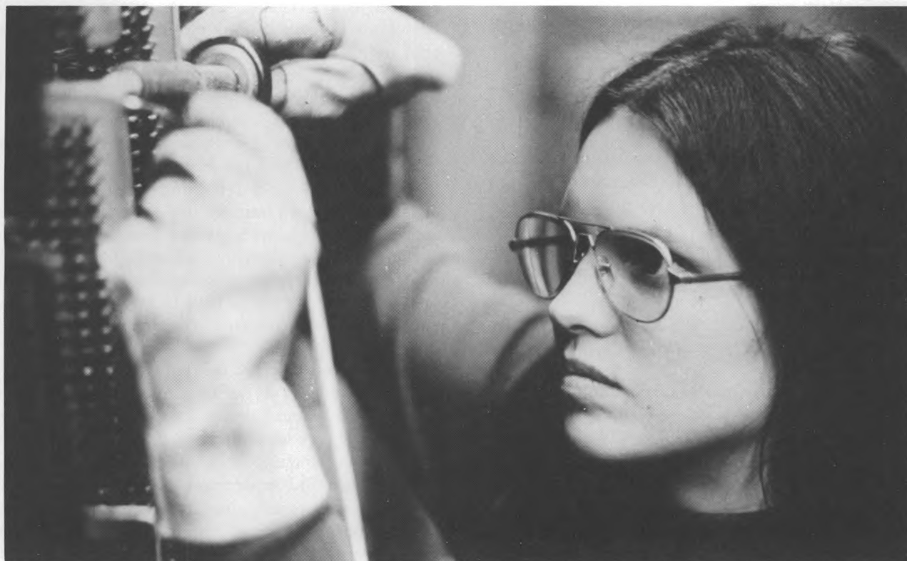
Good eye-hand coordination is needed to install telephone wiring.
