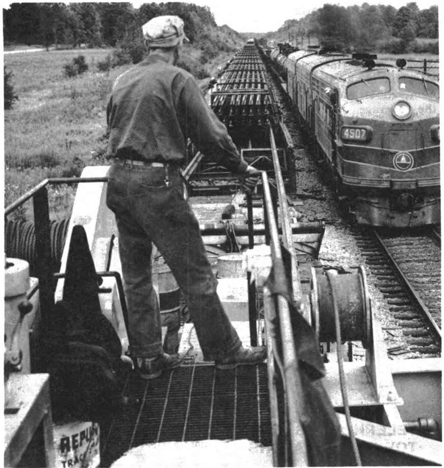
Track worker helps lay welded rail.
