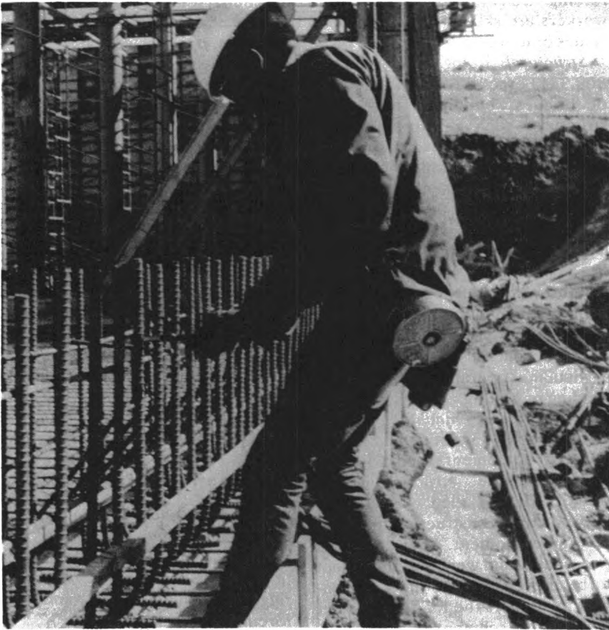
Reinforcing iron worker ties metal rods in place.
