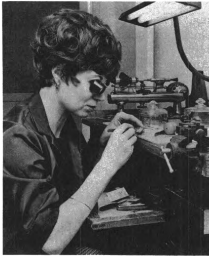
Watch repairer uses eye loupe to examine watch movement.
