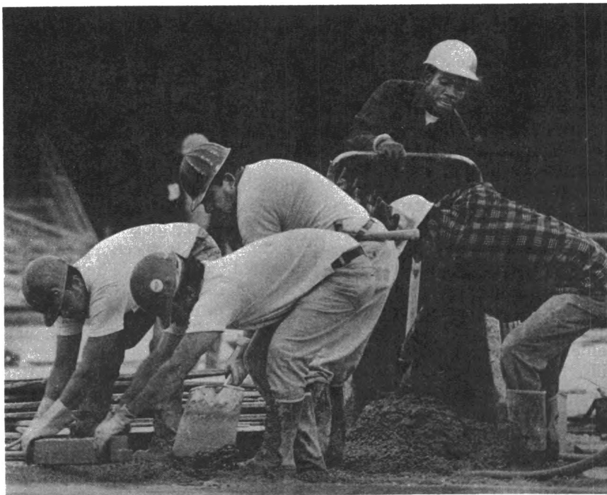
Cement masons prepare concrete floor.
