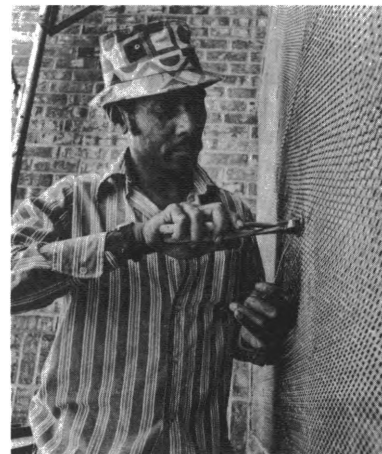
Lather wire-ties metal lath.
