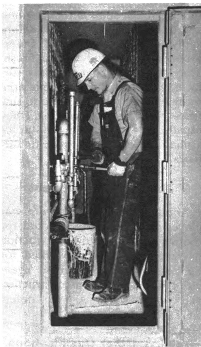
Plumbing is one of the highest paying building trades.
