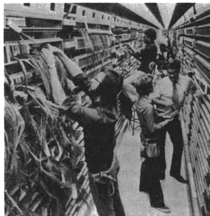
Central office equipment installers wire a new distribution frame and switching equipment.
