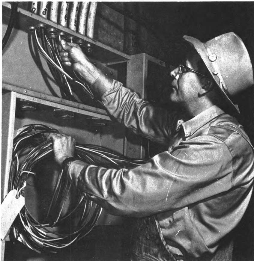
Electrician installs wiring.
