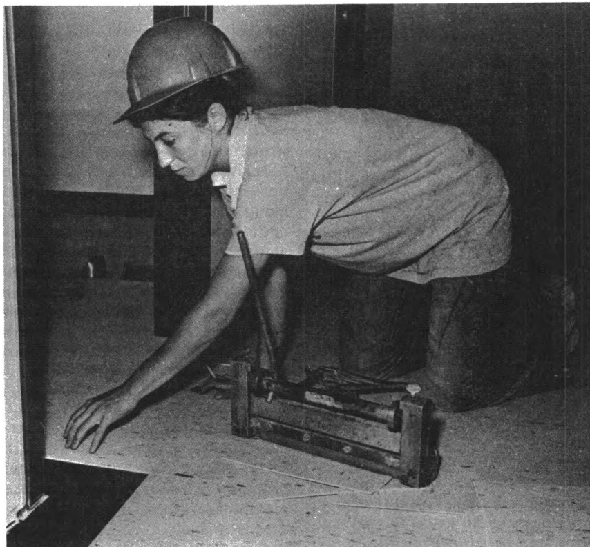
Floor covering installer lays resilient tile.
