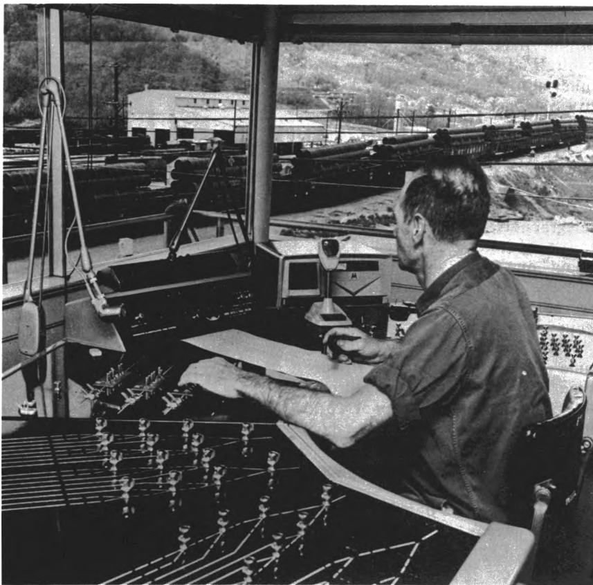
Glass enclosed towers provide tower operators with a clear view of the track below.
