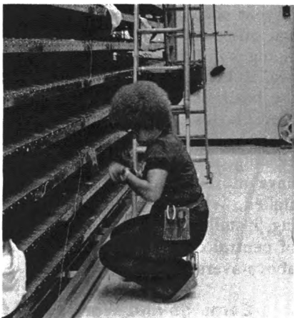
Frame wirer makes connection for new telephone.
