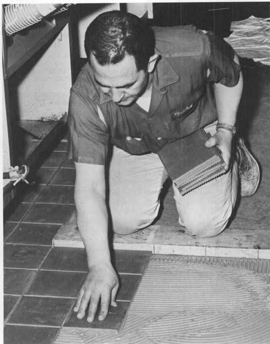
Tilesetter installs ceramic floor tile.
