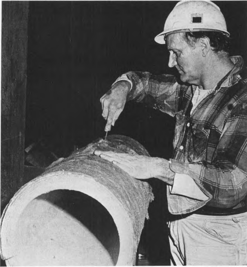
Asbestos worker cuts insulating material.
