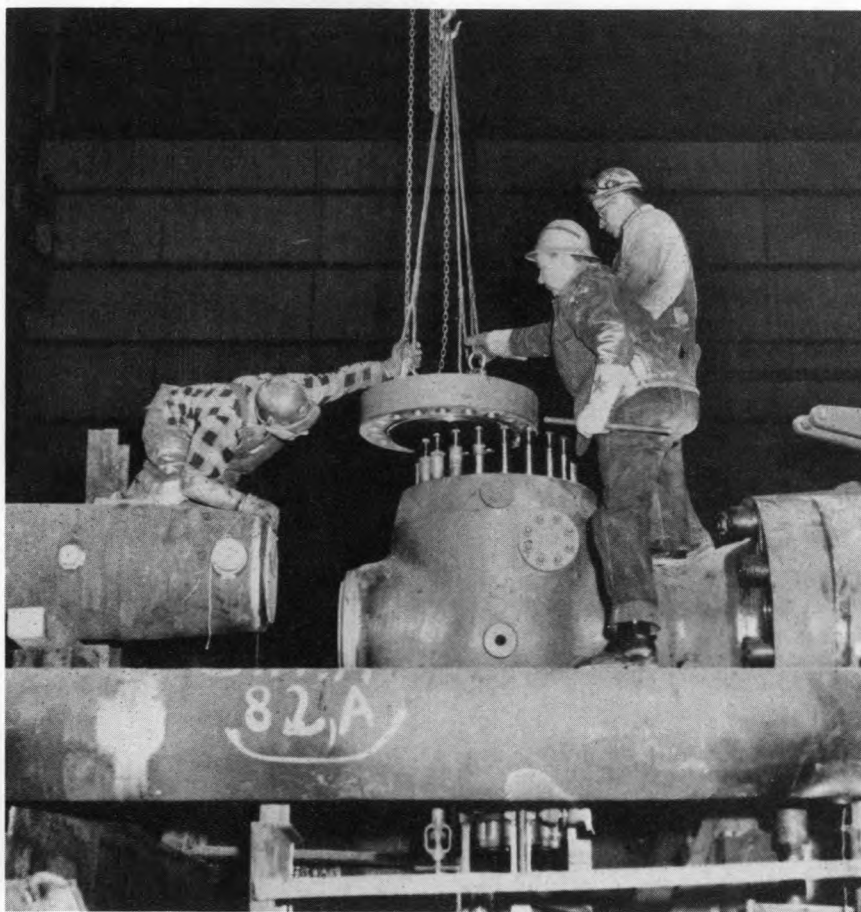
Millwrights move machinery into place.
