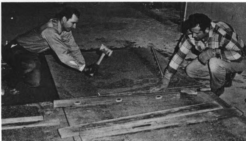
Stone masons adjust stone floor panel.
