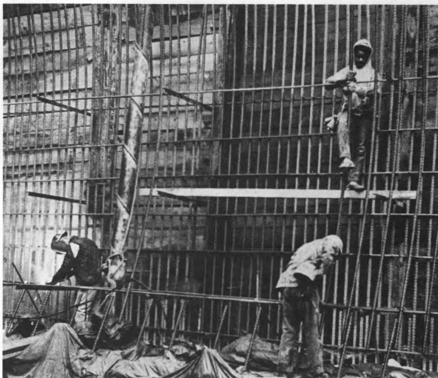
Rodmen position reinforcing bars.
