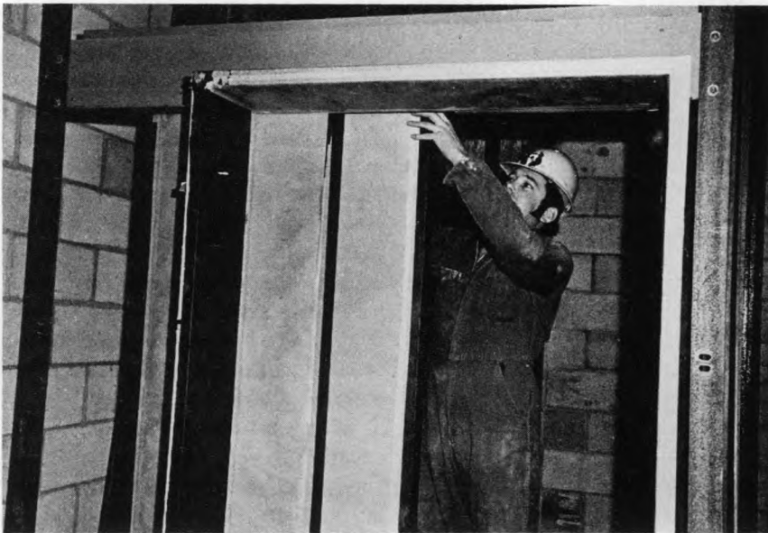
Elevator constructor adjusts door.
