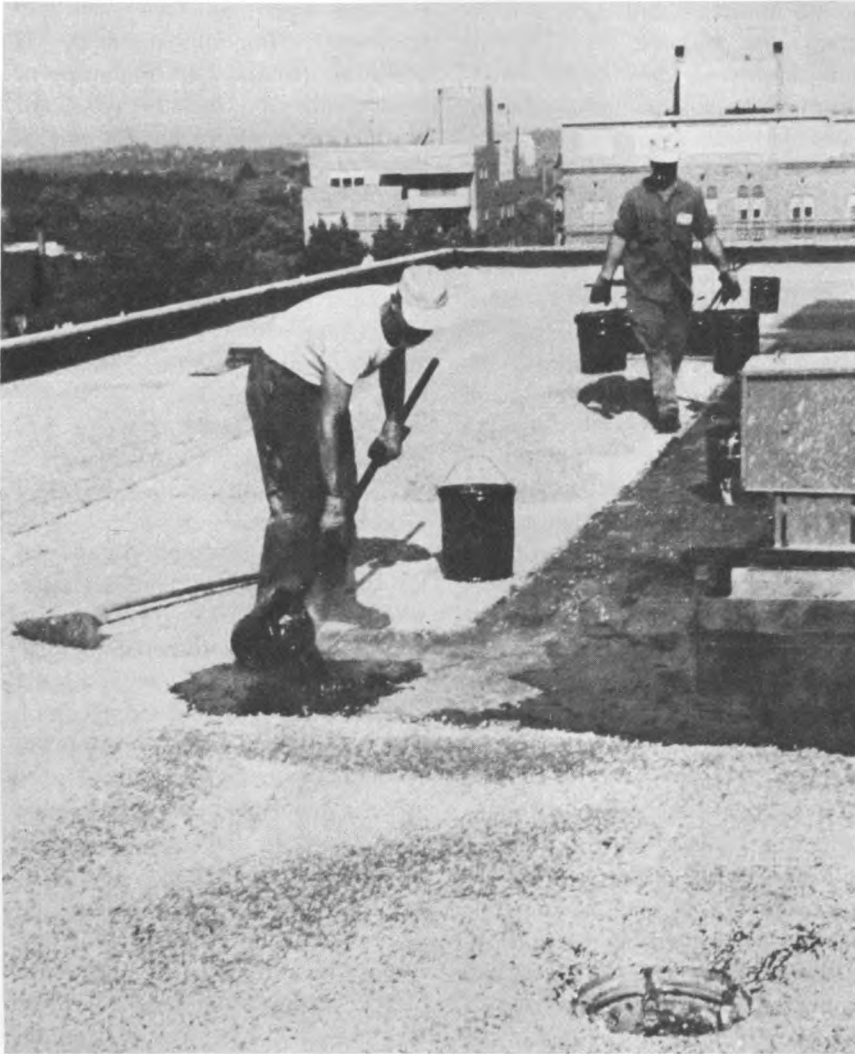
Roofers apply tar prior to spreading gravel.
