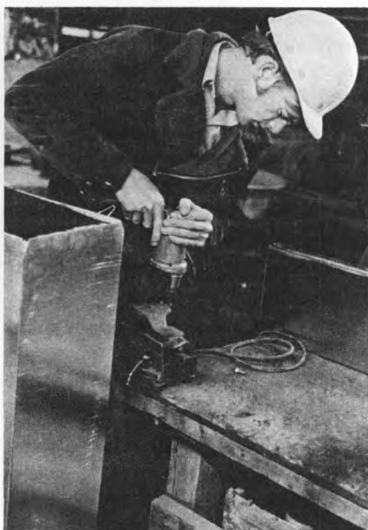
Sheet-metal worker drills sheeting.
