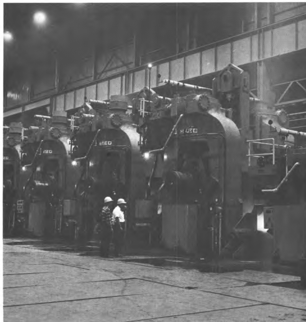
14. Hot Strip Mill Finishing Stands
