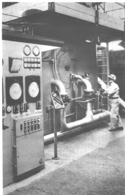
Stationary fireman opens valve in gas line to burner.
