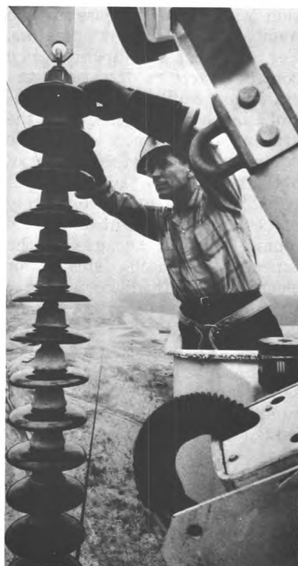
Lineman works on transmission line.
