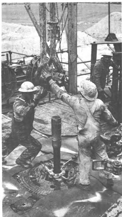
Roughnecks prepare to change drilling bit.
