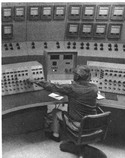
Operator at instrument console controls generating plant.
