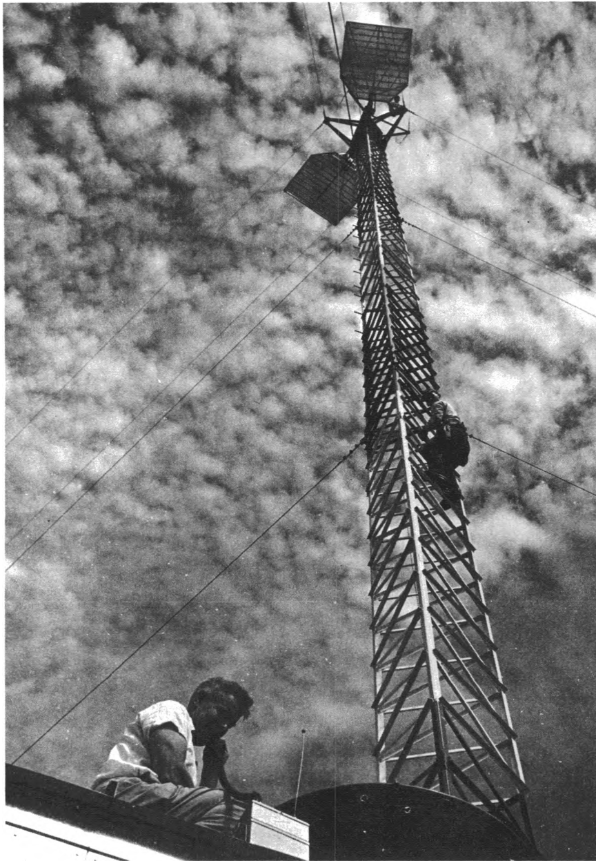
Signal maintainers check signal strength of repeater station.
